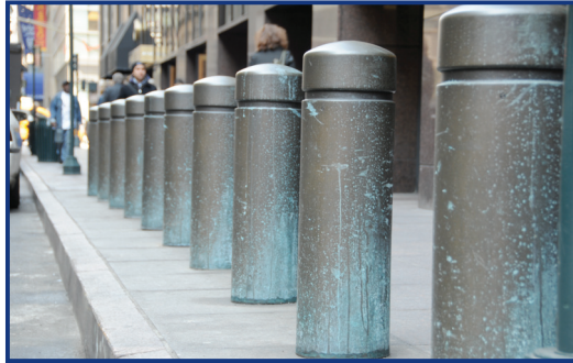
K-rated bollards create a hard perimeter.
